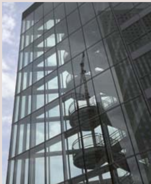
▲ Figure 5. Façade of a building made of glass with titanium dioxide nanoparticles
