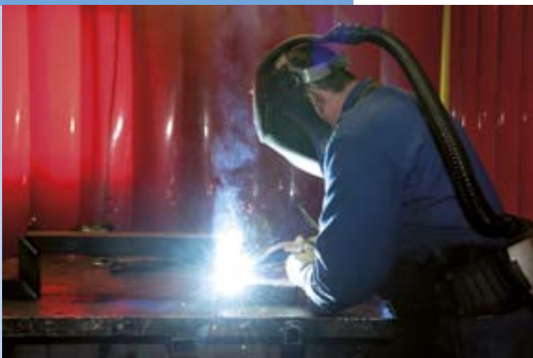
◀ Figure 9. Arc welding operation
