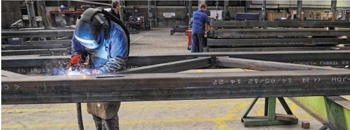
Welding operation on a metallic structure with a blowtorch
