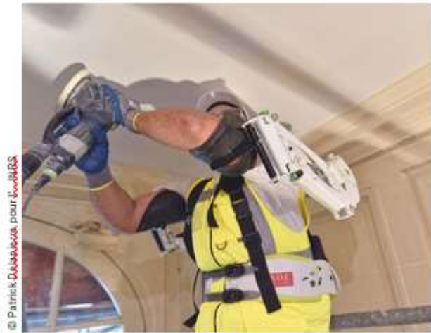
The development of a tailor-made exoskeleton enabled the Paris company Stuc. & Staff to limit the risk of MSDs at its renovation worksites for a specific task – sanding of ceilings.
