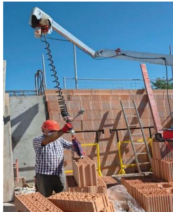
Bricklayers using a manipulator arm to move bricks
