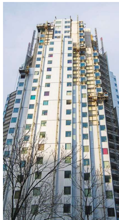
An exterior insulation project for a high-rise building.
