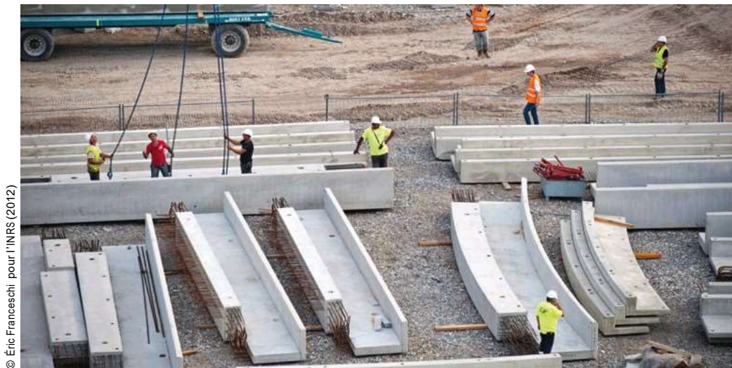
A prefabrication zone for stands at the Nice stadium construction site where several players operate at the same time.
