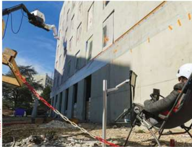
A painting robot for buildings developed by the Paintup company .
